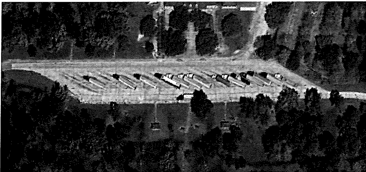
Figure 16: The Existing Parking Configuration at the Hancock County Welcome Center
