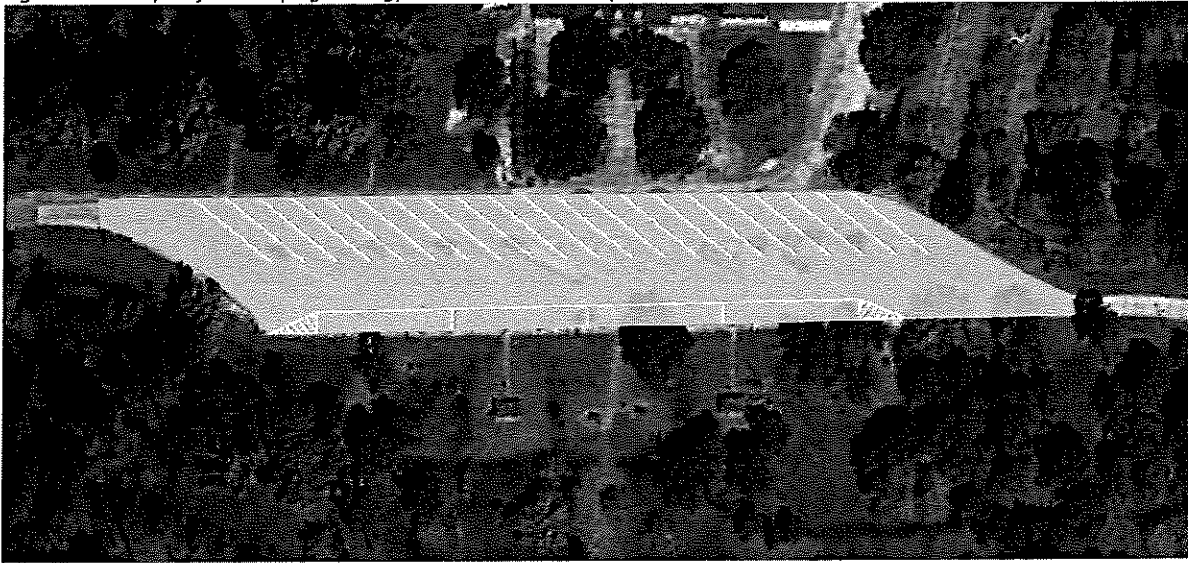
Figure 17: Example of a Restriping Strategy at the Hancock County Welcome Center
